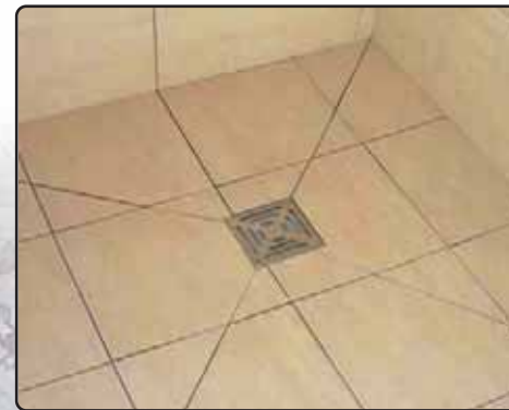
Varme Offset Shower Tray (pre-grout). Tiles cut to follow pre-made fall.
